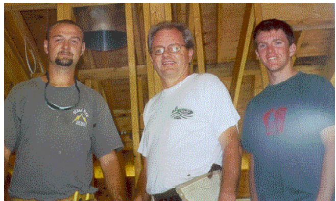
Ray Poudrier, center, of OceanView Electric, with assistance from Paul, left and Jeff, right, completed the electrical wiring for the Habitat home site on Cochran Ave. in Whitesboro last Fall.
